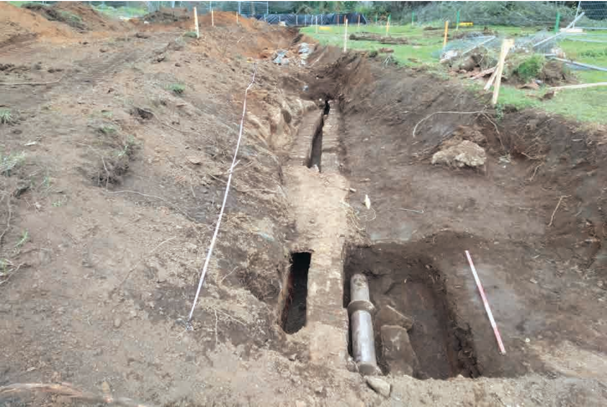
Figure 10. Feature 1, brick drain, and Feature 10, ceramic drainage pipe (scale = 1 m).
