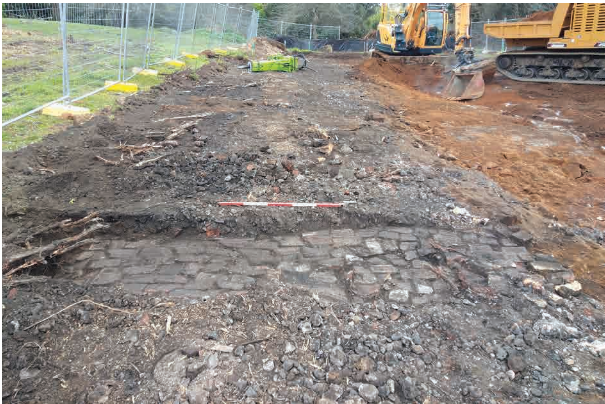
Figure 19. Section of Feature 7, brick paved road or driveway, looking west (scale = 1 m).
